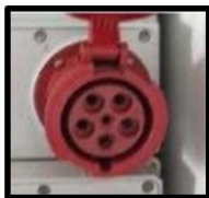
1 CEE 63A 5p 400V (Triple Phase 50Hz)
